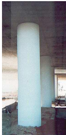
Fig. 9 Application of Carbon Fibre Column Wrap and completed Carbon Fibre Wrap [3]; Fig.10 Application of Carbon Fibre Column Wrap and completed Carbon Fibre Wrap [3]
