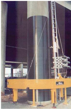
Fig. 9 Application of Carbon Fibre Column Wrap and completed Carbon Fibre Wrap [3]; Fig.10 Application of Carbon Fibre Column Wrap and completed Carbon Fibre Wrap [3]
